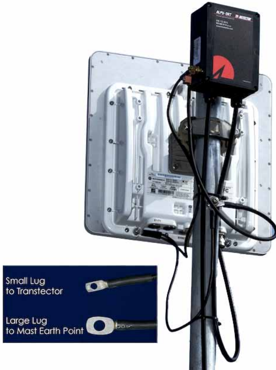
Figure 112 - Upper Grounding Configuration
