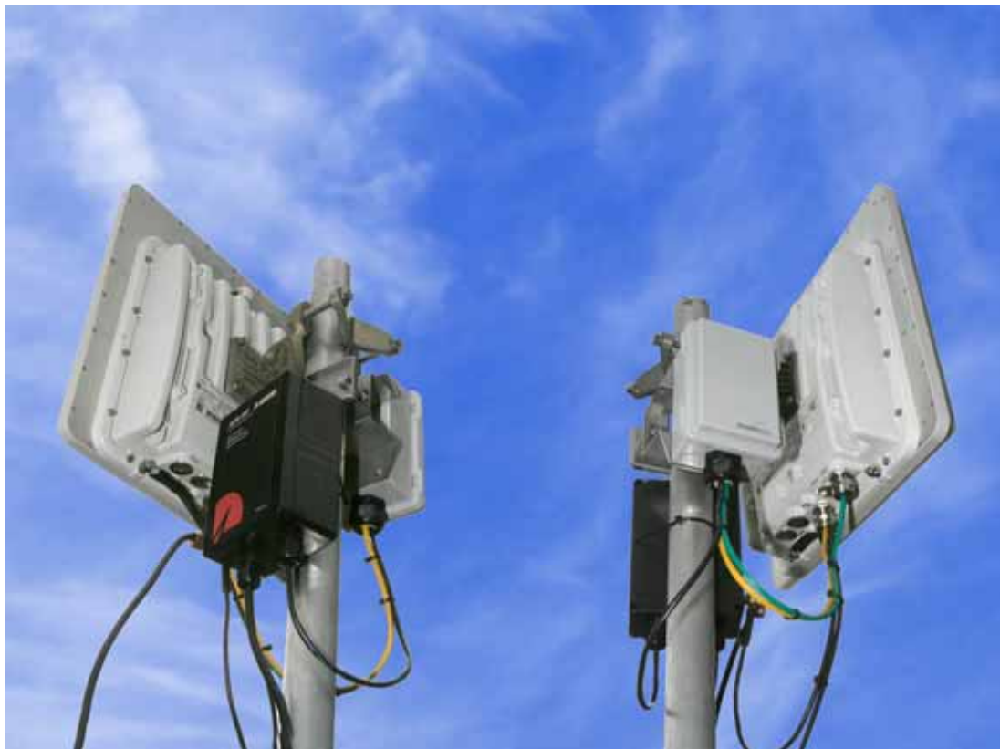
Figure 130- GPS Synchronization Unit Complete Installation
