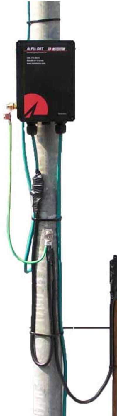
Figure 113 - Lower Grounding Configuration
