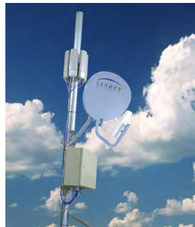
Figure 13: CMM2 pole-mounted
